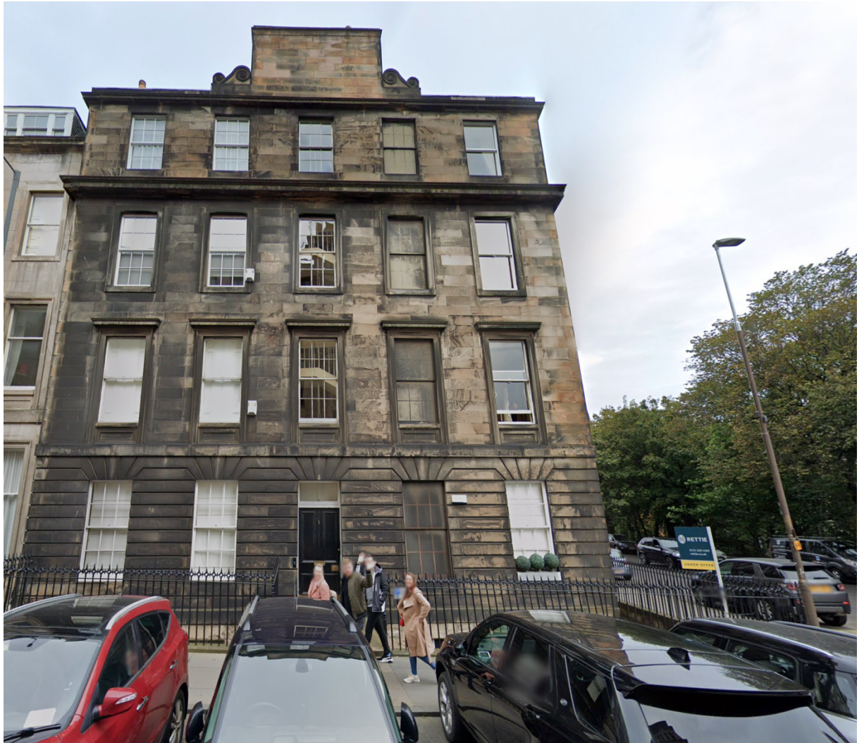
Photo 7 – View of the 4-storey tenement at 1 Cambridge Street in which the application site is located at basement level
