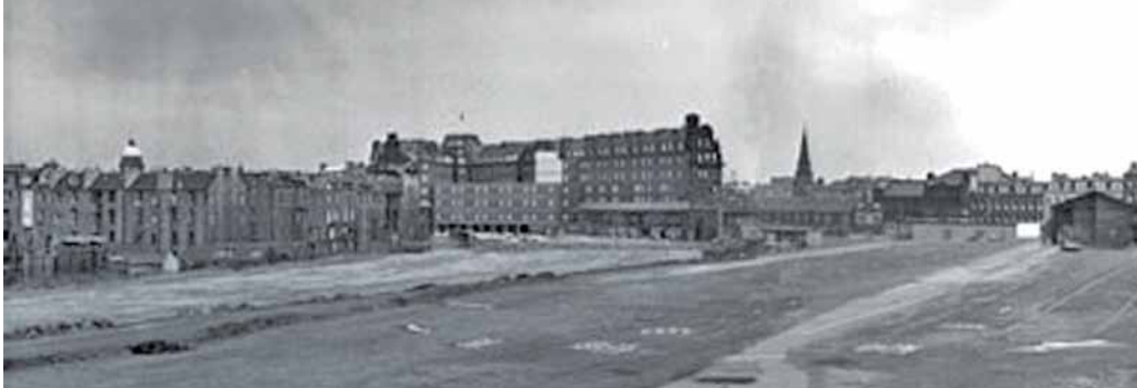
Lothian Road Goods Yard
