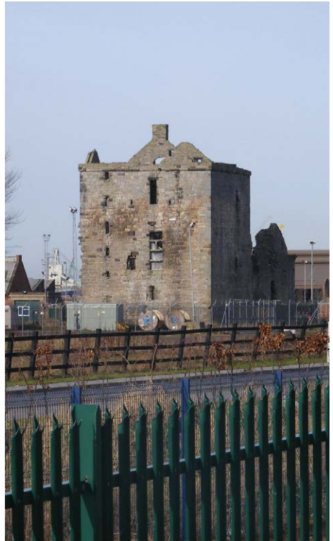
Rosyth Castle, Fife. Once located on an island in the River Forth, the site was incorporated into the naval dockyards in the 20th century resulting in significant change to the scheduled monument's original setting. Any changes, including enhancement, need to be considered against the current setting.
