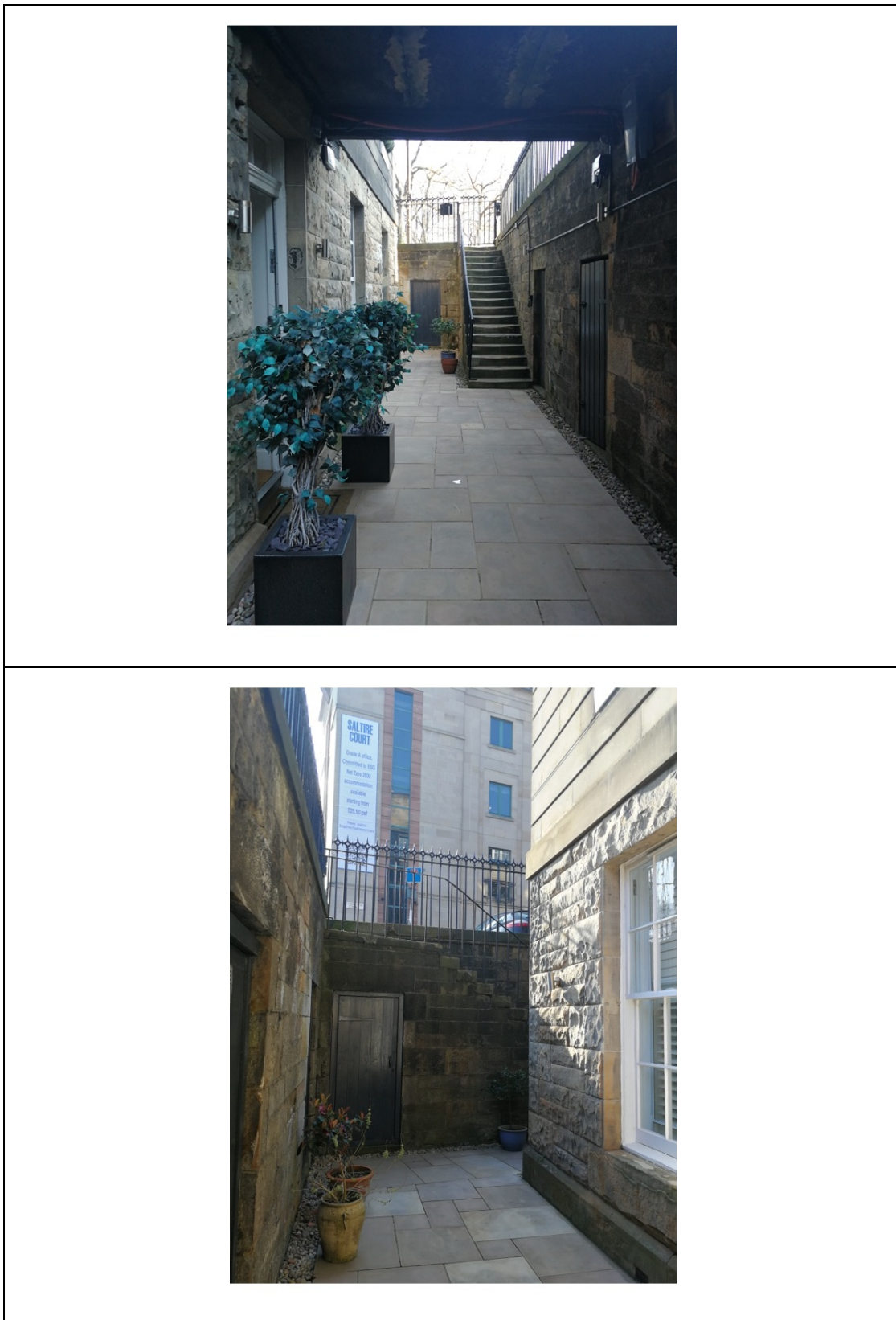
Photo 10 – View of the application site from basement level
