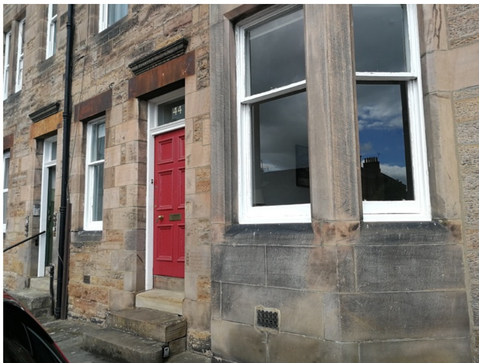
Photo 1a – Application site and established residential/mixed-use area of the Morningside Conservation Area: Jordan Lane
