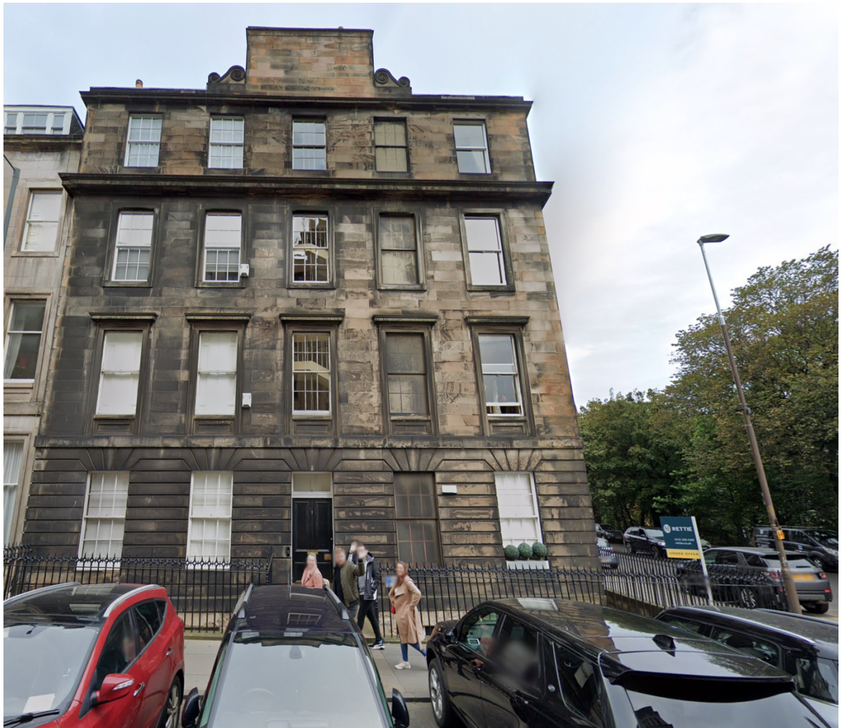
Photo 7 – View of the 4-storey tenement at 1 Cambridge Street in which the application site is located at basement level
